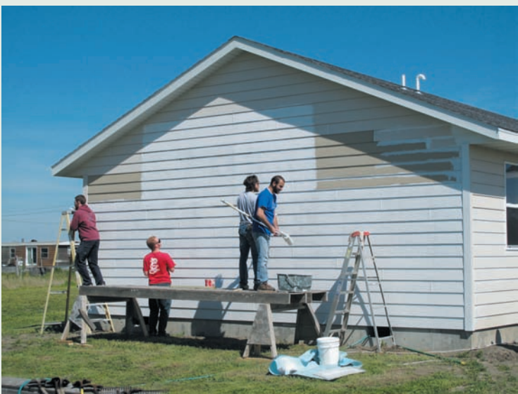
Our paint team at work.
