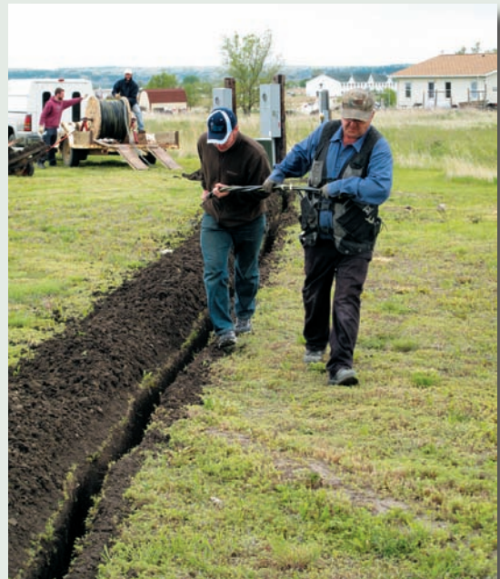
Pulling the main service wire to the house.
