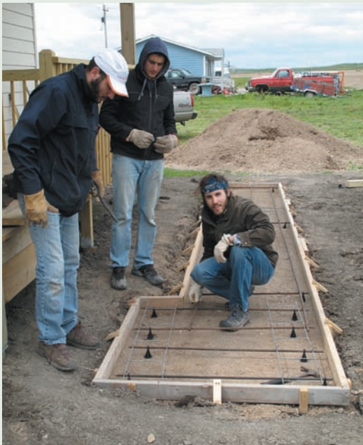
Doing form work for the front sidewalk.
